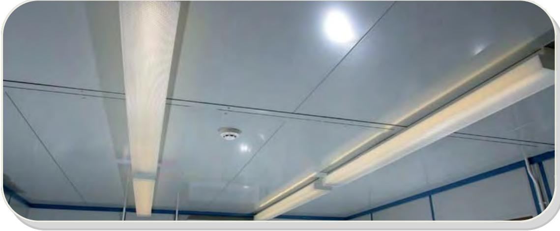
Spans above 2980 require an integrated beam which has a colour matched cover to the underside.
