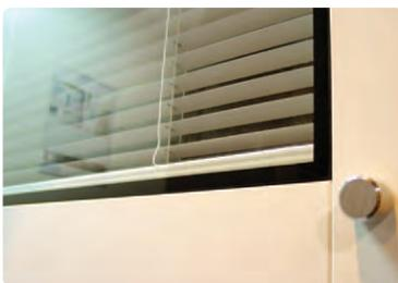
Flush glazing is supplied as standard. This reduces the number of ledges and junctions, giving an improved functionality and aesthetic appearance.
